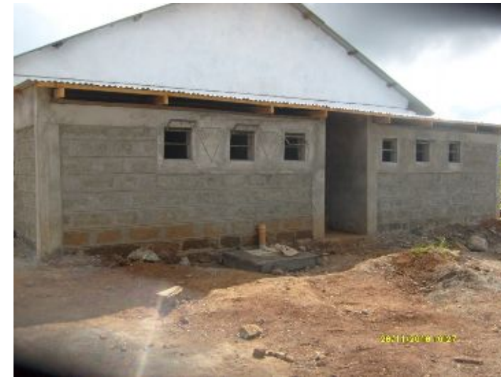
The boy's bathrooms and toilets block.
